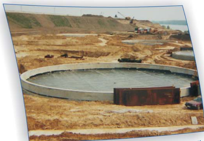
Platforma petrolieră Giurgiu-lești Constructor: TMUCB
